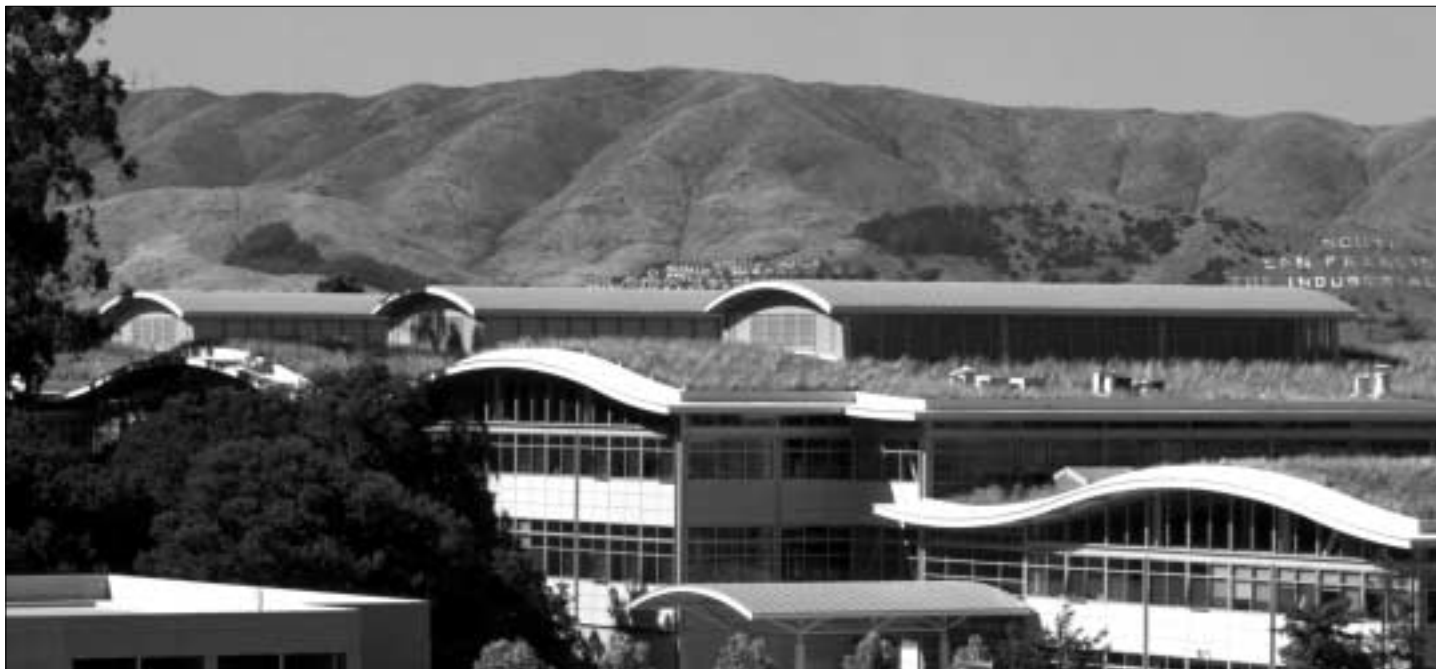
The roof of 901 Cherry (offices of Gap, Inc.) recreates the native habitat of grasses and wild flowers. Its form derives from the surrounding landscape. © William McDonough + Partners
