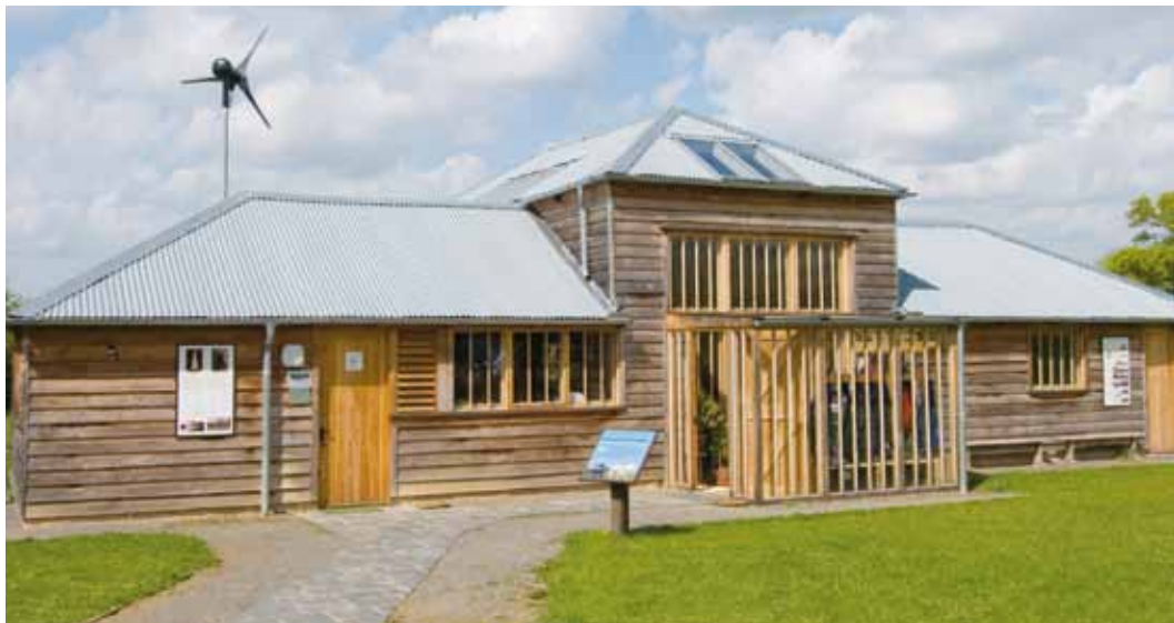
Figure 5.2: The Foundry – carbon neutral refurbishment of a former traction engine shed.
